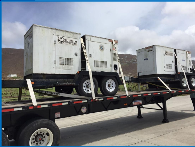
US Army Corps Generators headed to Guam after Typhoon Mawar
